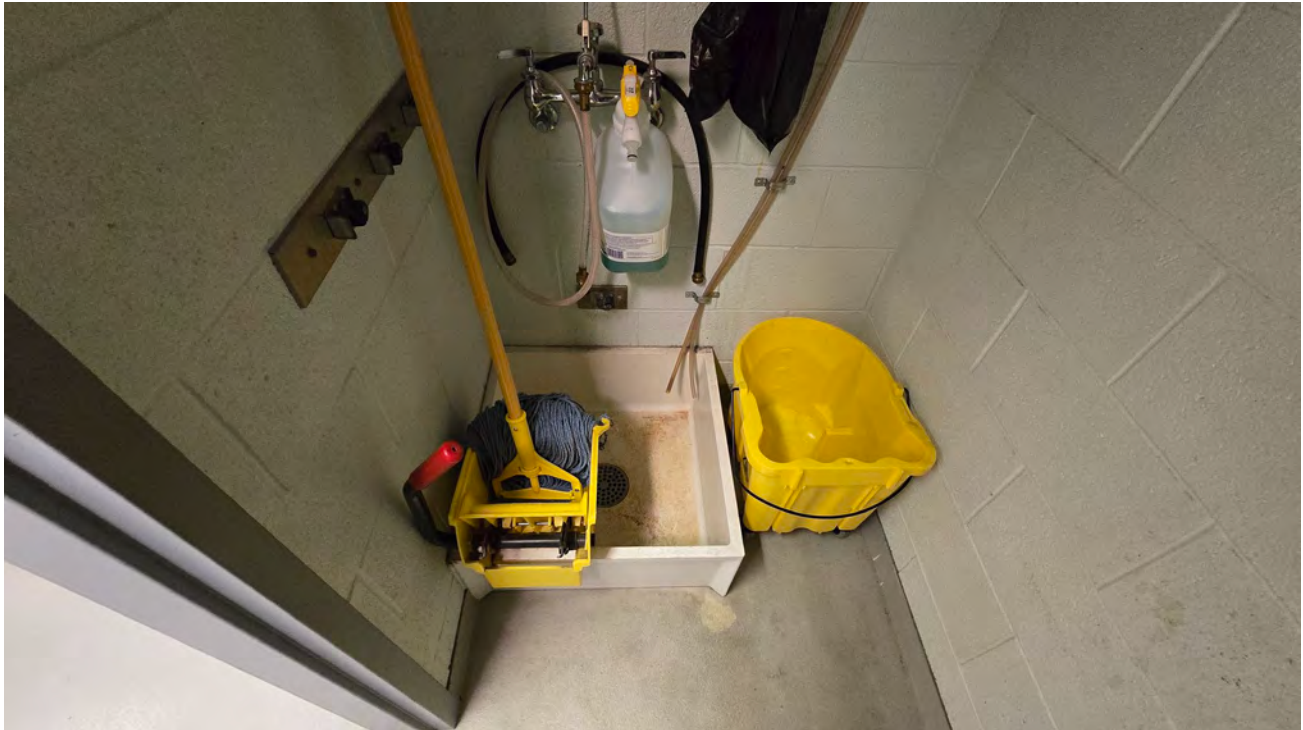
Photograph # 21: Janitorial closet on second floor with drain.
