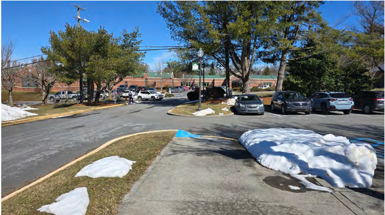
Photograph # 7: Looking northeast from northeast building entrance.
