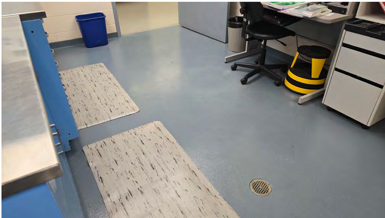
Photograph # 29: Second floor laboratory equipped with floor drain connected to acid dilution tank.
