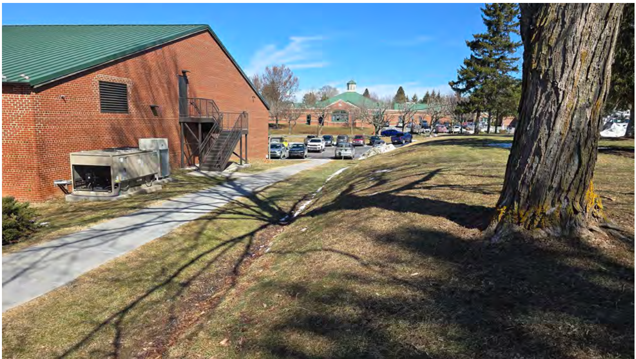
Photograph # 12: Looking northeast along western side of site.
